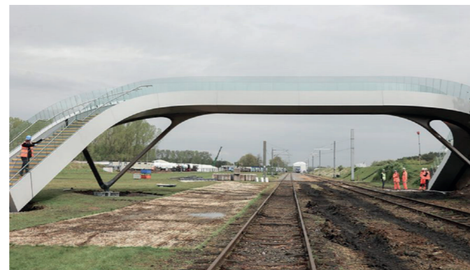
Network Rail prototype of innovative low-cost modular footbridge
